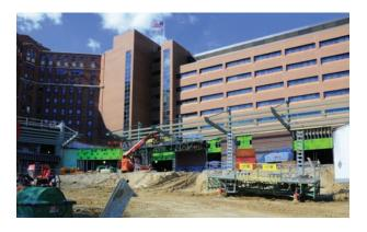
fireproofing of the structural steel and metal roof deck can be completed. Soon the structure will see the installation of the brick and stone masonary. Finally, the aluminum curtain wall and new glass will be complete by the middle of November.
